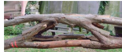
Fig. 3: Construction components made from naturally grown, unprocessed wood
